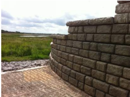
Figure 7-2: Redi-Rock wing wall and Armorflex (photo reproduced with permission of CPM Group)
